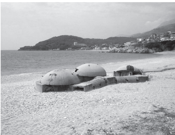
Figure 6. Picture of bunkers realised after year 1990, where can be observed well the filling of their communicator hallway by gravel and sand. Its high was 1.20 m (according to Stefa E., et. al. 2009).
