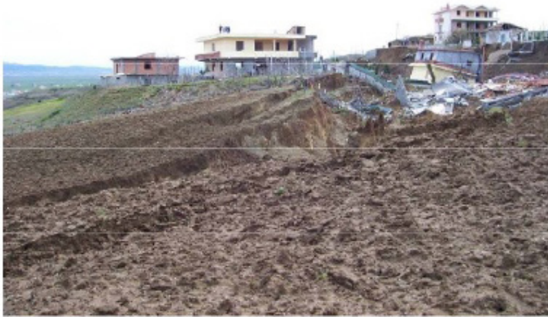
Figure 3. Soil cracks where the landslide has happened, in the study area
